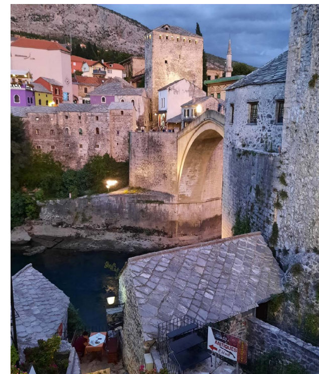
A view of the now rebuilt bridge just before dusk
